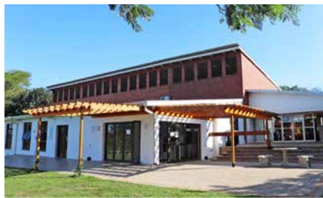
New school shop (left) and new coffee shop (right)
